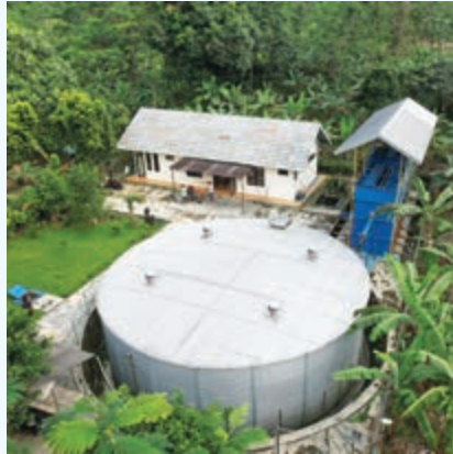
Water Treatment Plant (WTP)
